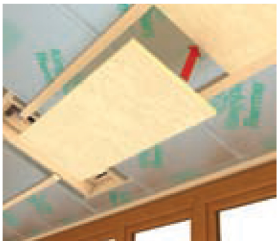
Install insulation between batten
