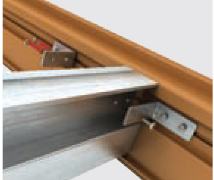
Fix rafters to ringbeam
