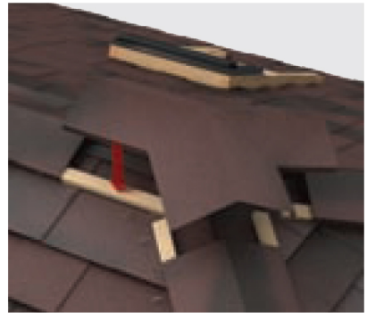
Fix rafter cap and ridge
