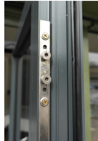
Espag Locking Mechanism
